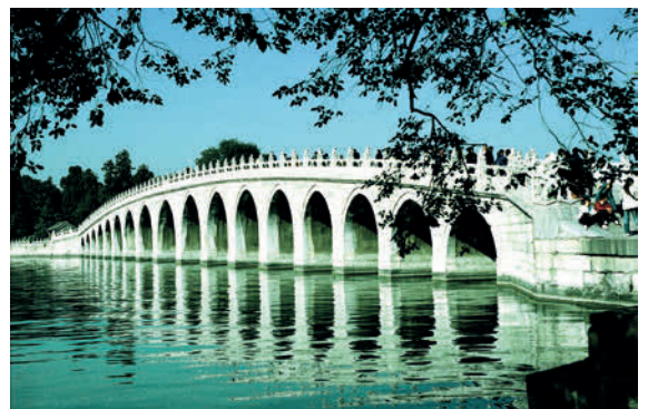
Fig.2 Seventeen-Arch Bridge in Beijing 北京十七孔橋
