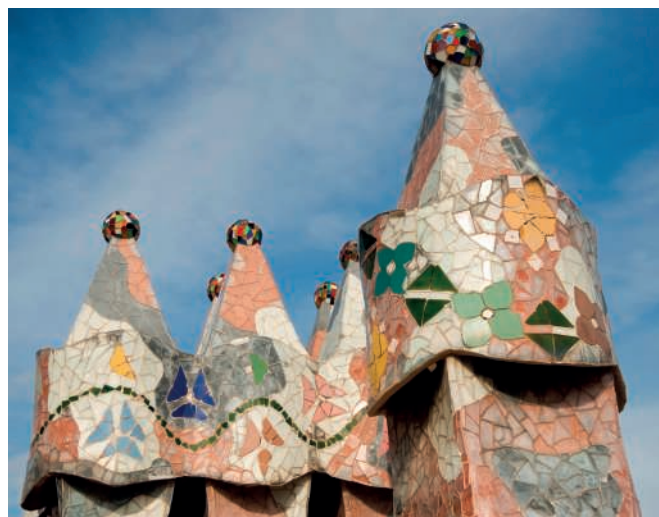
Antoni Gaudí, Casa Batlló Chimneys, Barcelona, redesigned in 1904. Photo: GM Photo Images / Alamy Stock Photo.
